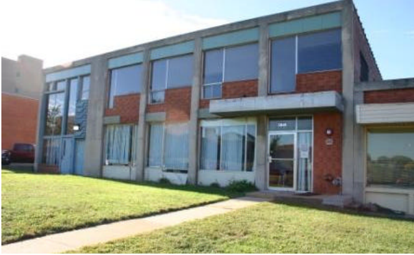
3840 Washington - office/storage space
